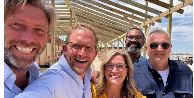
Lancium's Expansion Project Lancium & Crusoe broke ground on the first facility located in Lancium's Clean Campus
